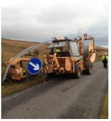
Moleplough of 4 way direct in ground sub duct on Jura
